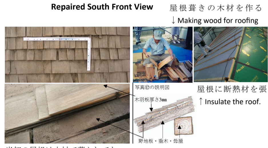
当初の屋根は木材で葺かれてた The original roof was pitched with wood.
